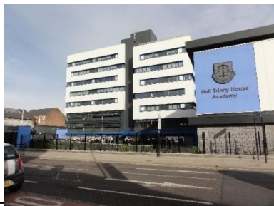
Above: Derek Crothall Building in 2013 (when it was part of Trinity House School) Below right: Brewery House, The Maltings
