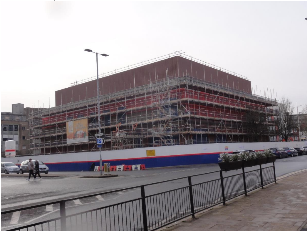
Community Diagnostics Centre 4.1.25
