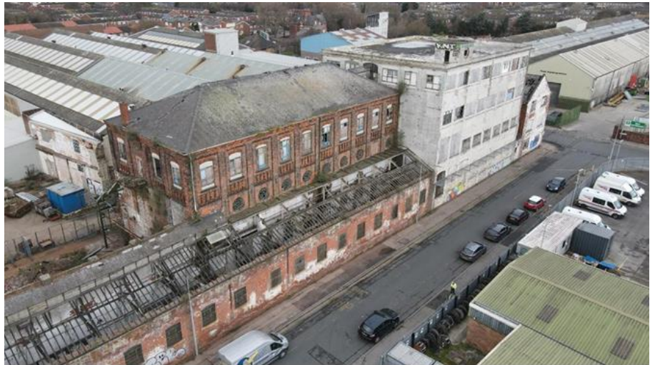
Hennebique Building & Bottom Shop – Caroline St Elevations
