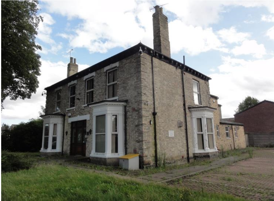
John Symons House, Park Row (a cul-de-sac on the west side of Park Street) 19.8.23
