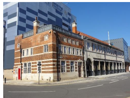
Former Central Fire Station, now Steam Studios
