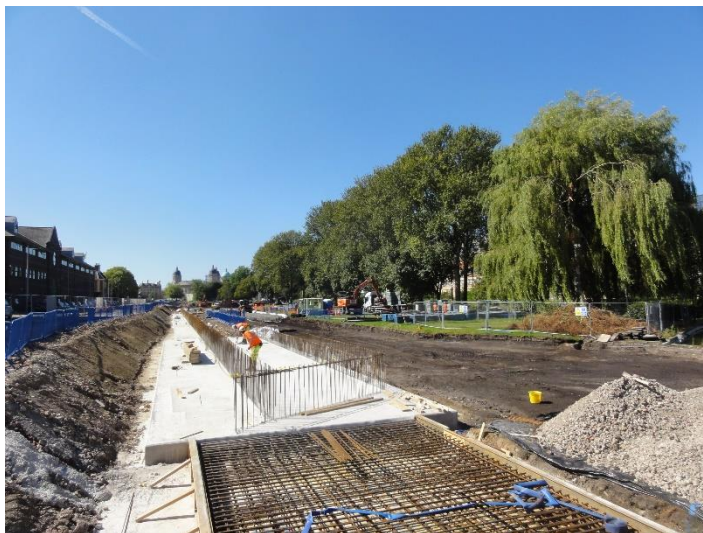
Work in progress in Queen's Gardens 5.9.23
