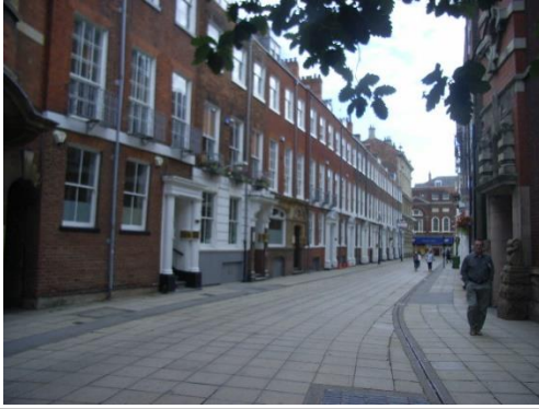
Above left: 2 Parliament St (first on the left) right: John Symons House, Park Row
