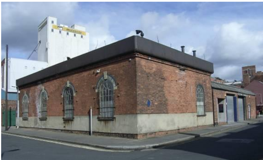
Hull Hydraulic Power Station, Machell Street
