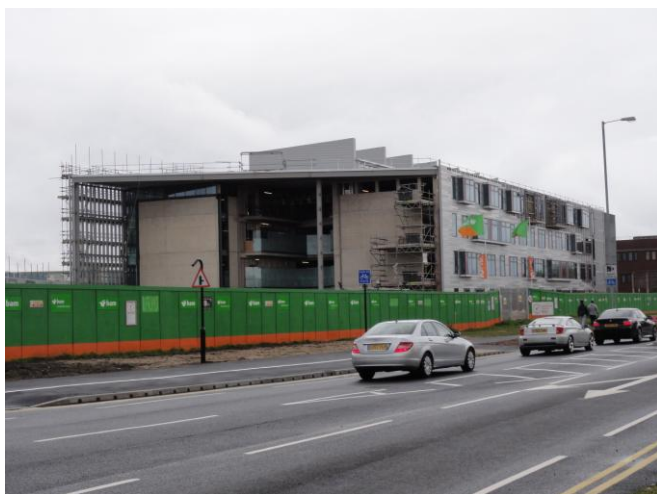
New Humberside Police HQ, Clough Road (Photo: JD Scotney)
