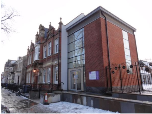
Western Branch Library, Boulevard – the new extension. (Photo: JD Scotney)
