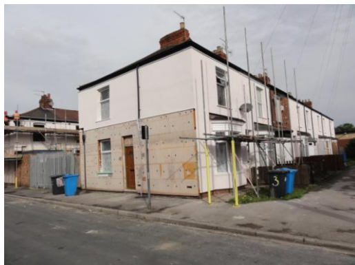
Houses being clad and refurbished in Albemarle St. (Photo: JD Scotney)
