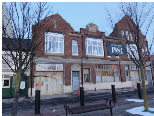
Hesslegate Buildings (Photo: JD Scotney)
