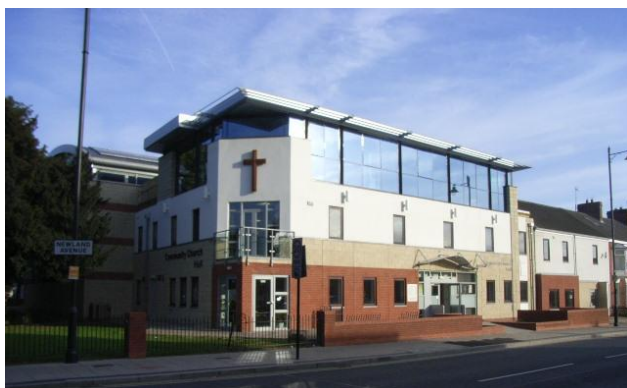
Hull Community Church, with building work complete. (Photo: J D Scotney)
