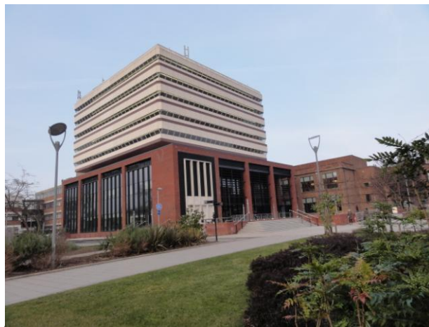
Brynmor Jones Library – south and west façades in 2015. Photo: JD Scotney
