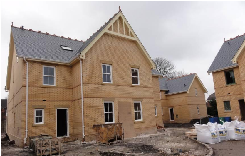
Above: Newland Homes original orphanage houses (1890s) Below: Ashcourt's new student accommodation (2014). Note the matched detail in bricks, barge boards, roof slates and barge boards. (Photos: JD Scotney)
