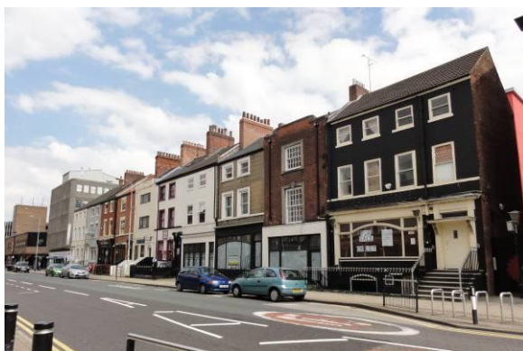
62/64 (right foreground) to 72 (the white building), George Street (Photo: JD Scotney)
