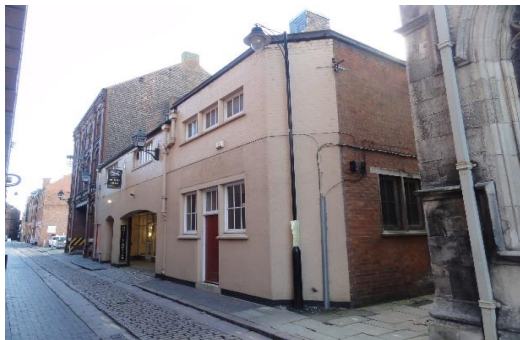
Right and below: 9-11 Chapel Lane
