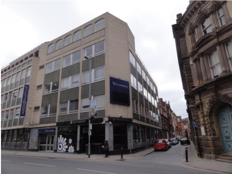
Sun Alliance Offices built 1968 and extended 1976
