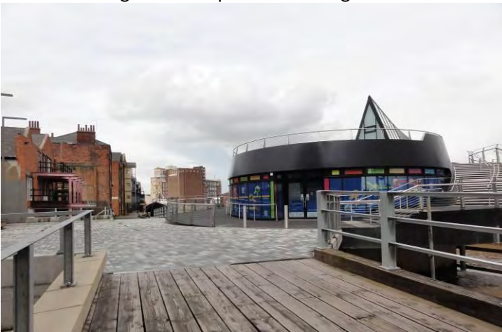
Scale Lane Bridge from the River Hull Walkway (Photo: J D Scotney)
