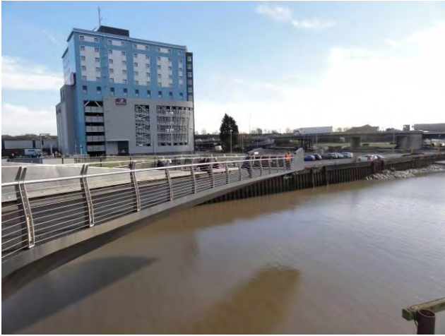
Scale Lane Bridge swinging open. (Photo J D Scotney)
