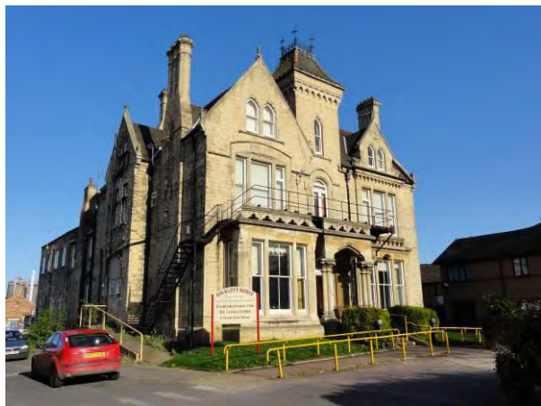
Rockcliffe House, Beverley Rd - former Blind Institute care home. (Photo: J D Scotney)
