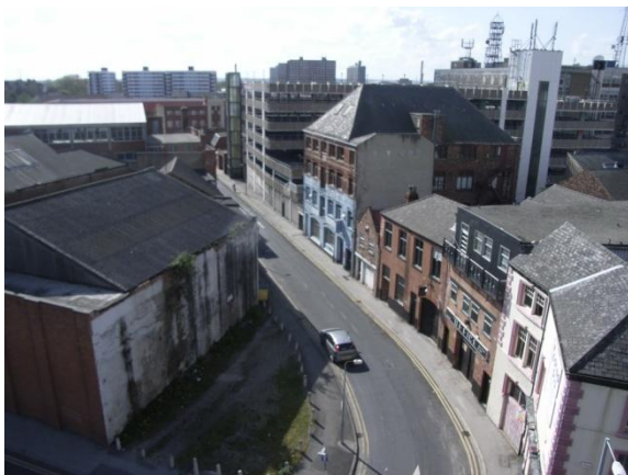
Roper St in 2009, viewed from Princes Quay car park: all demolished.. (Photo: JDS)
