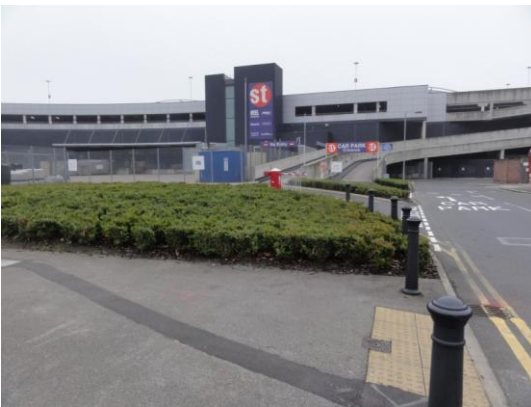
Entrance ramp to St Stephens car park in Canning Street (Photo: JDS)
