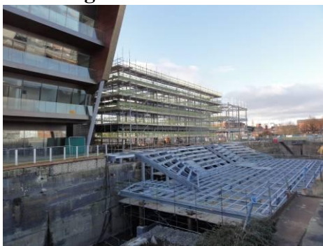
Central Dry Dock, arena and C4DI buildings. (Photo: JDS, 21.2.16)
