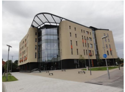
The Allam Medical Building
