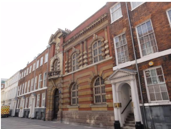
Parliament St - surviving sections of the old Central Police Station.
