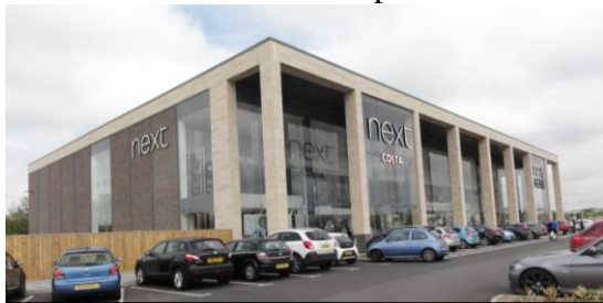
Next store at Kingswood
