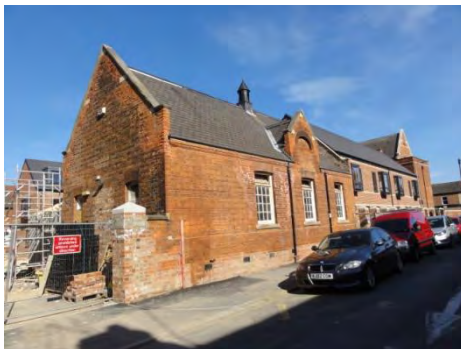
Part of former Newland Ave Primary School seen from Reynoldson St 25.9.18
