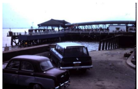
Above: The Pier in 1964 shortly before the upper deck was demolished. Below: the bridge and pontoon for loading people and vehicles onto New Holland ferries. (12.7.1981)
