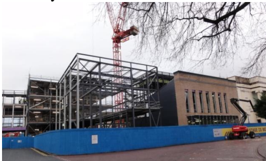
Ron Dearing UTC & New Theatre extension Kingston Square 8.12.16 (Photos: JDS)
