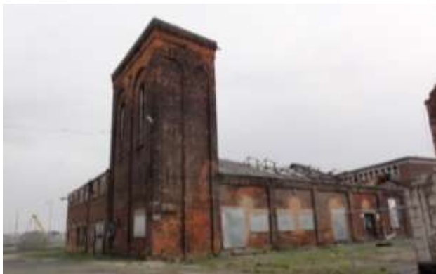
St Andrews Dock - hydraulic tower & pump house
