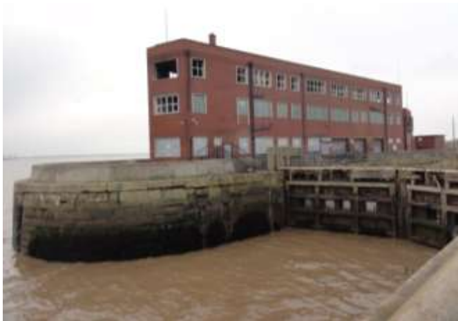
St Andrews Dock - Boston Building
