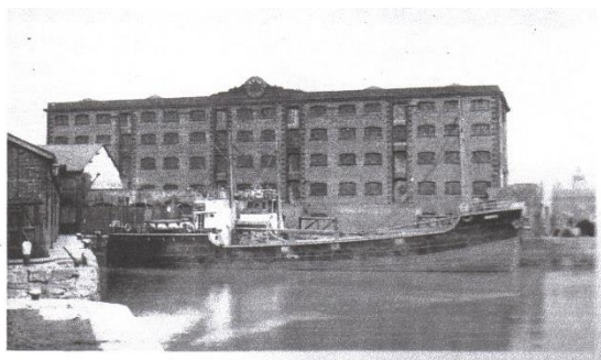
Above: Old Seven – from Humber Dock Right: side elevation
