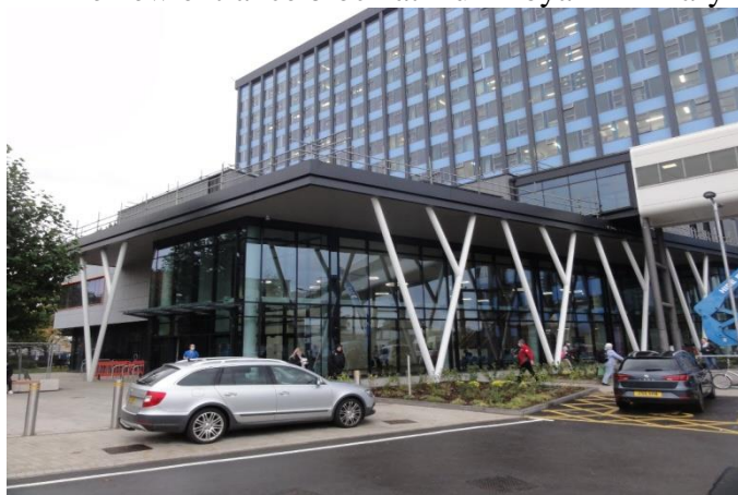
Hull Royal Infirmary new entrance, opened 18.10.22
