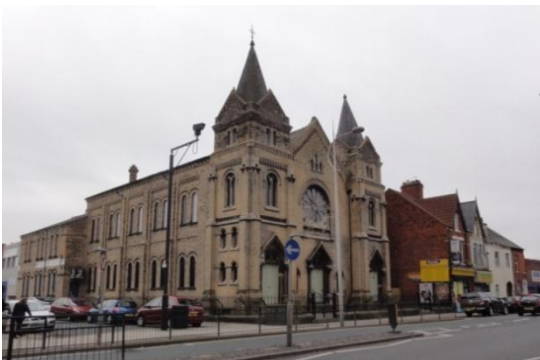
City Temple, Hessle Rd, showing former Sunday School block at the rear
