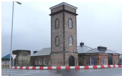
Alexandra Dock Hydraulic Pump House
