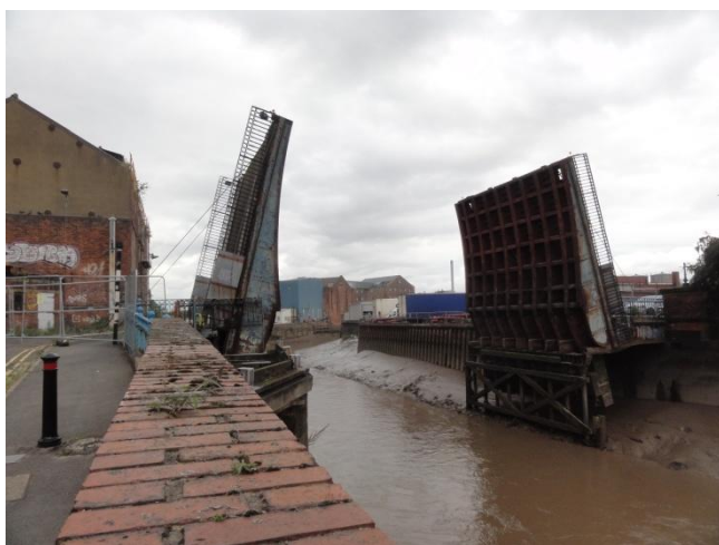
Scott Street Bridge
