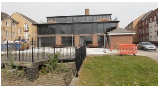
Victoria Dock winding house, 24.4.19
