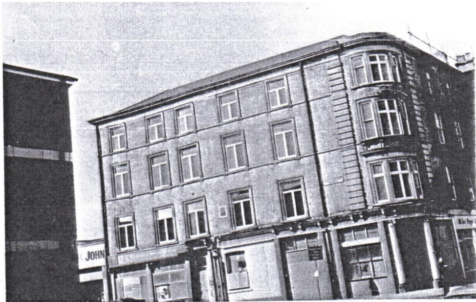
A sad loss: Wellington House (1850) demolished in 2015
